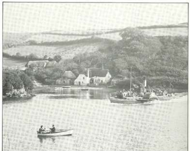
ILTON CASTLE IN SOUTH POOL CREEK – AN IDYLIC SETTING
