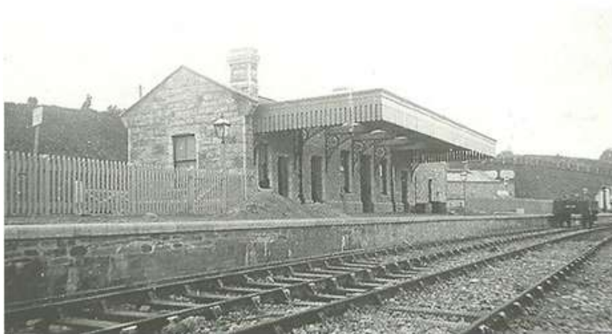
KINGSBRIDGE STATION SHORTLY BEFORE OPENING DAY ON 18 TH DECEMBER 1893
