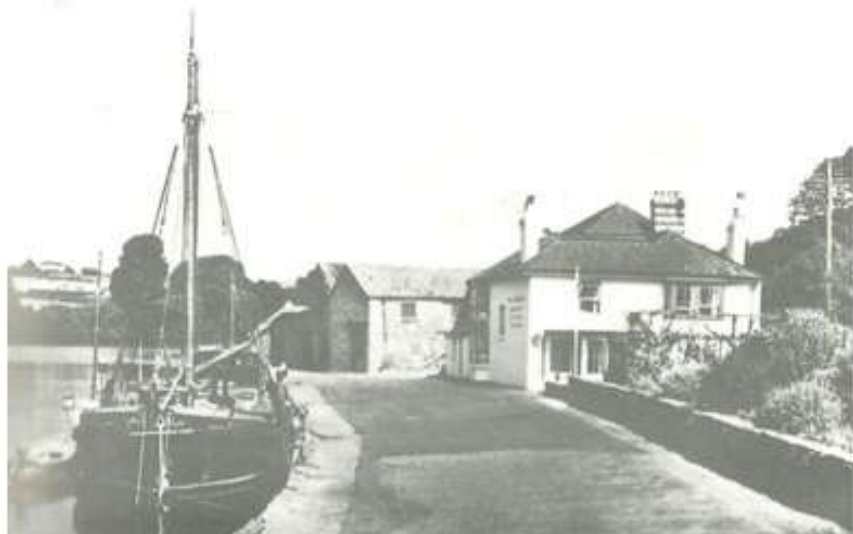
THE CRABSHHELL INN AT BOND'S QUAY FORMERLY NEW QUAY INN SET UP BY THE BOND FAMILY IN 1840'S WITH SAILING BOAT BERTIE
